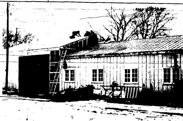
Workers are shown here putting a roof on the expansion to the welding and machine shop at Carroll, owned by Morris Sandahl. The building has been expanded 49 feet to the west and is 30 feet wide.
